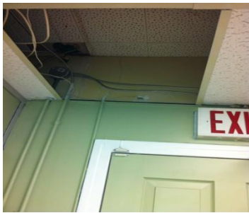
Figure 3: TLR- Missing ceiling tiles, leaky ceiling
