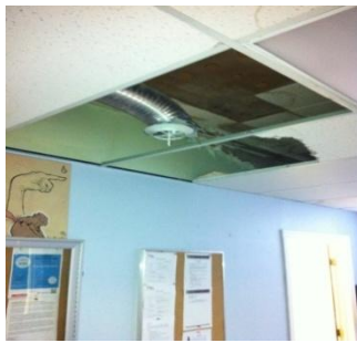
Figure 3: TLR- Missing ceiling tiles, leaky ceiling
